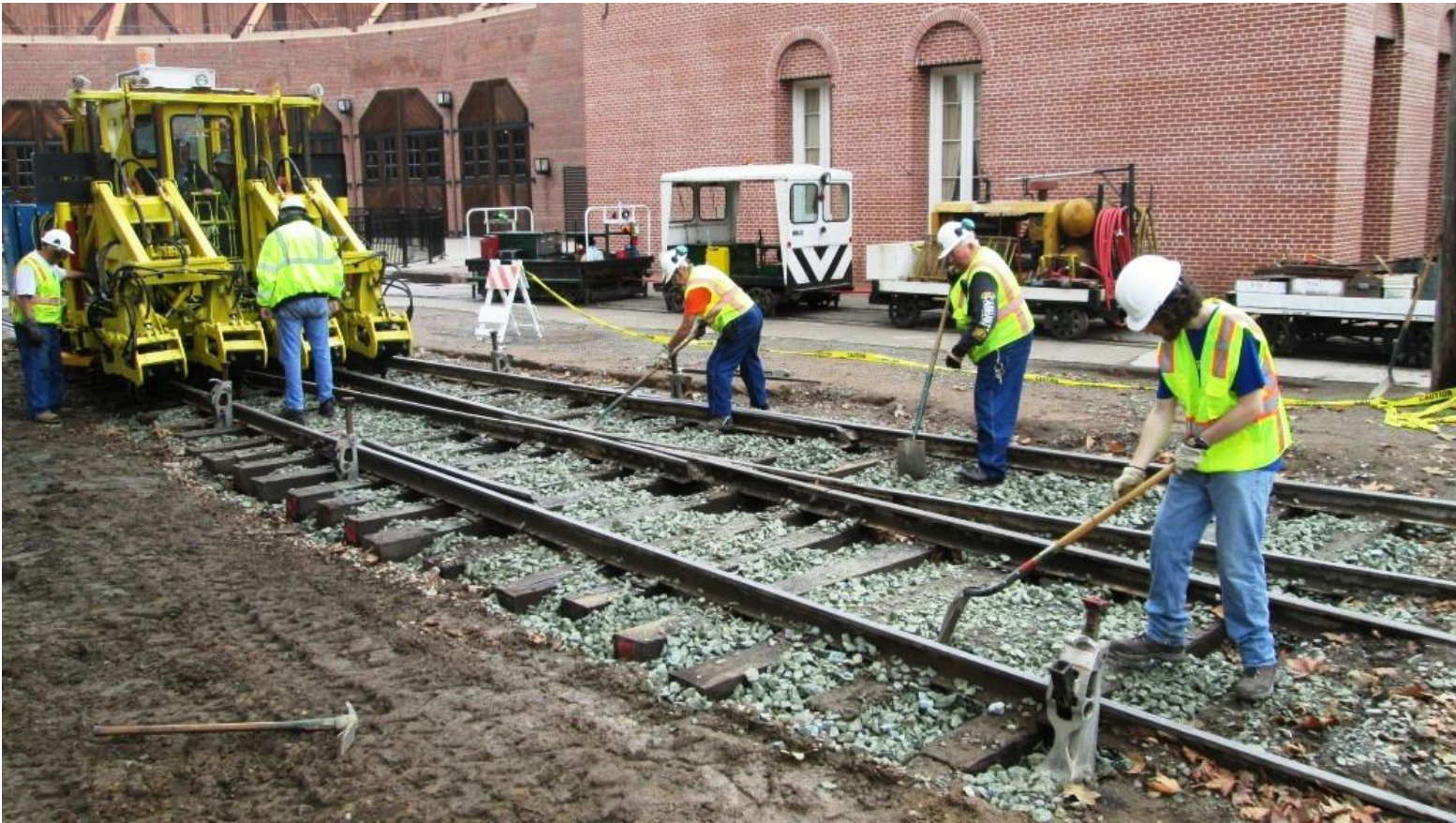
At the Turnout, Clem and Alan work with Chris and Pam in the Tamper while Ed, Harry, and Matt spread-out the rock
