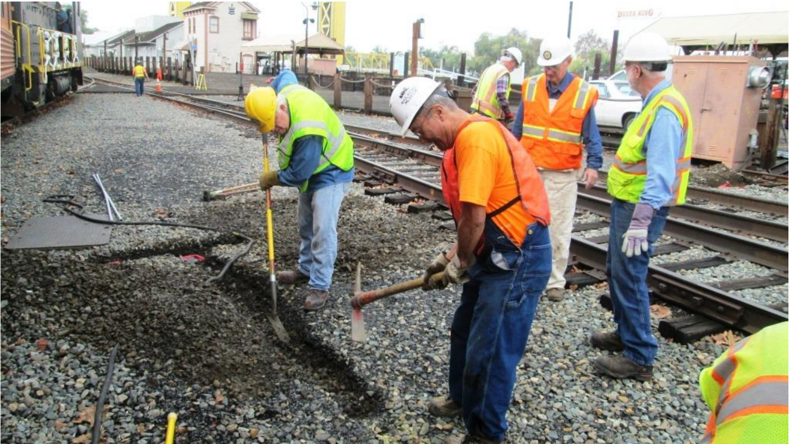
Jim and John keep on trenching
