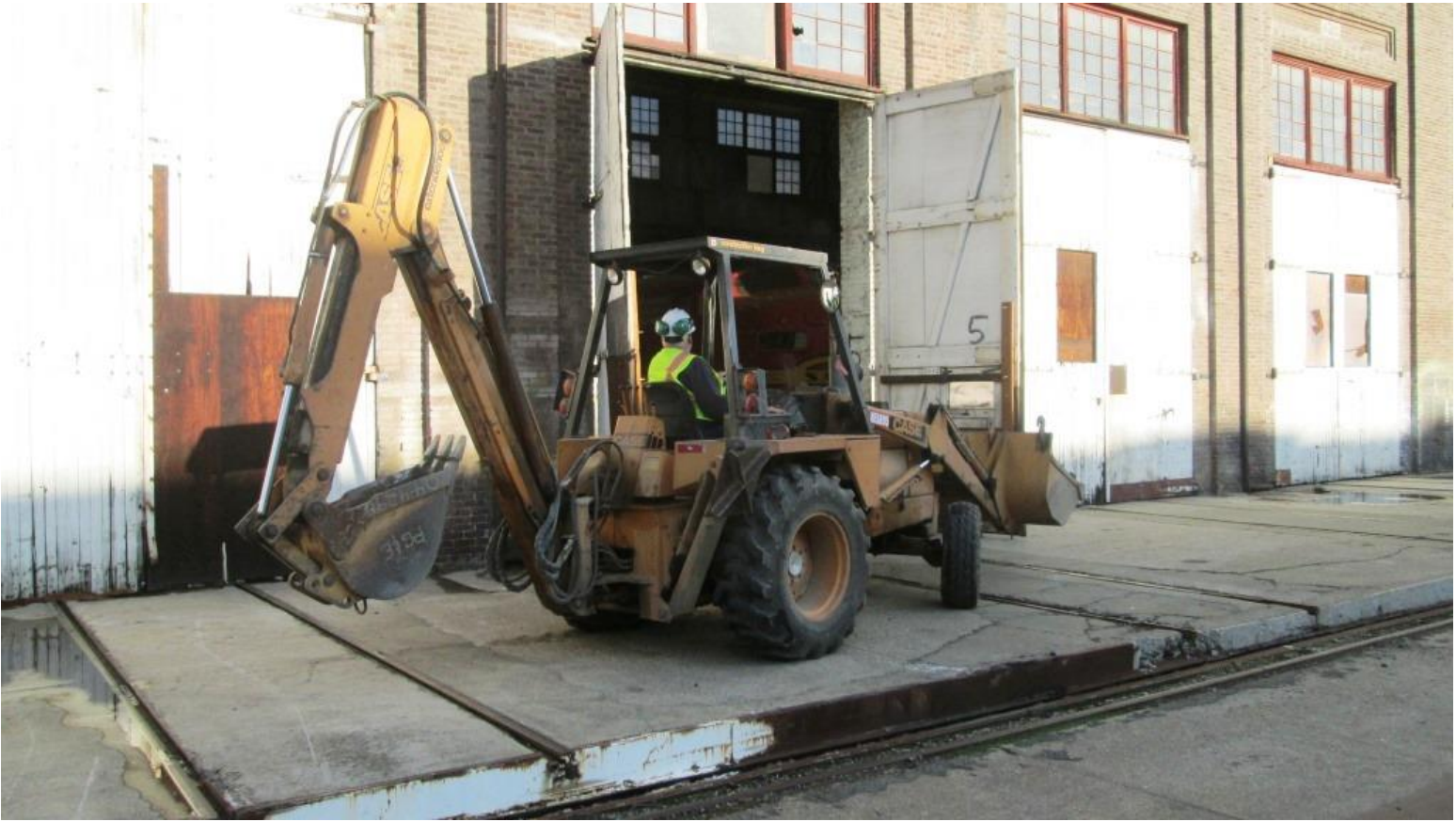
Harry takes the back-hoe into the Erecting Shop
