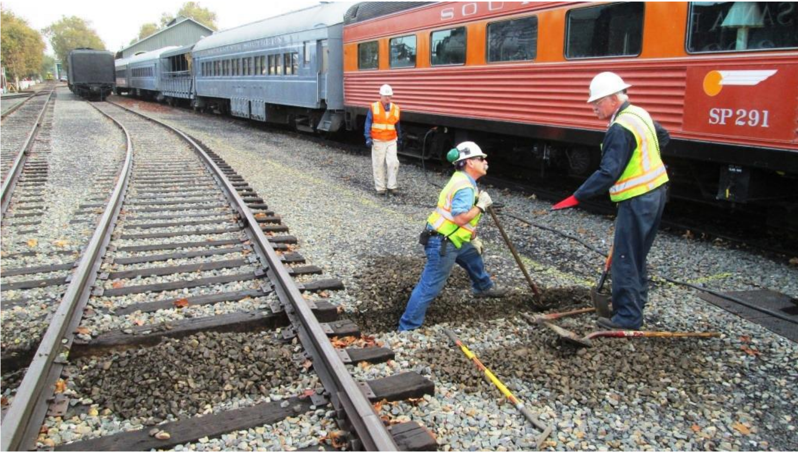
Joe and Gary confer about trench depth
