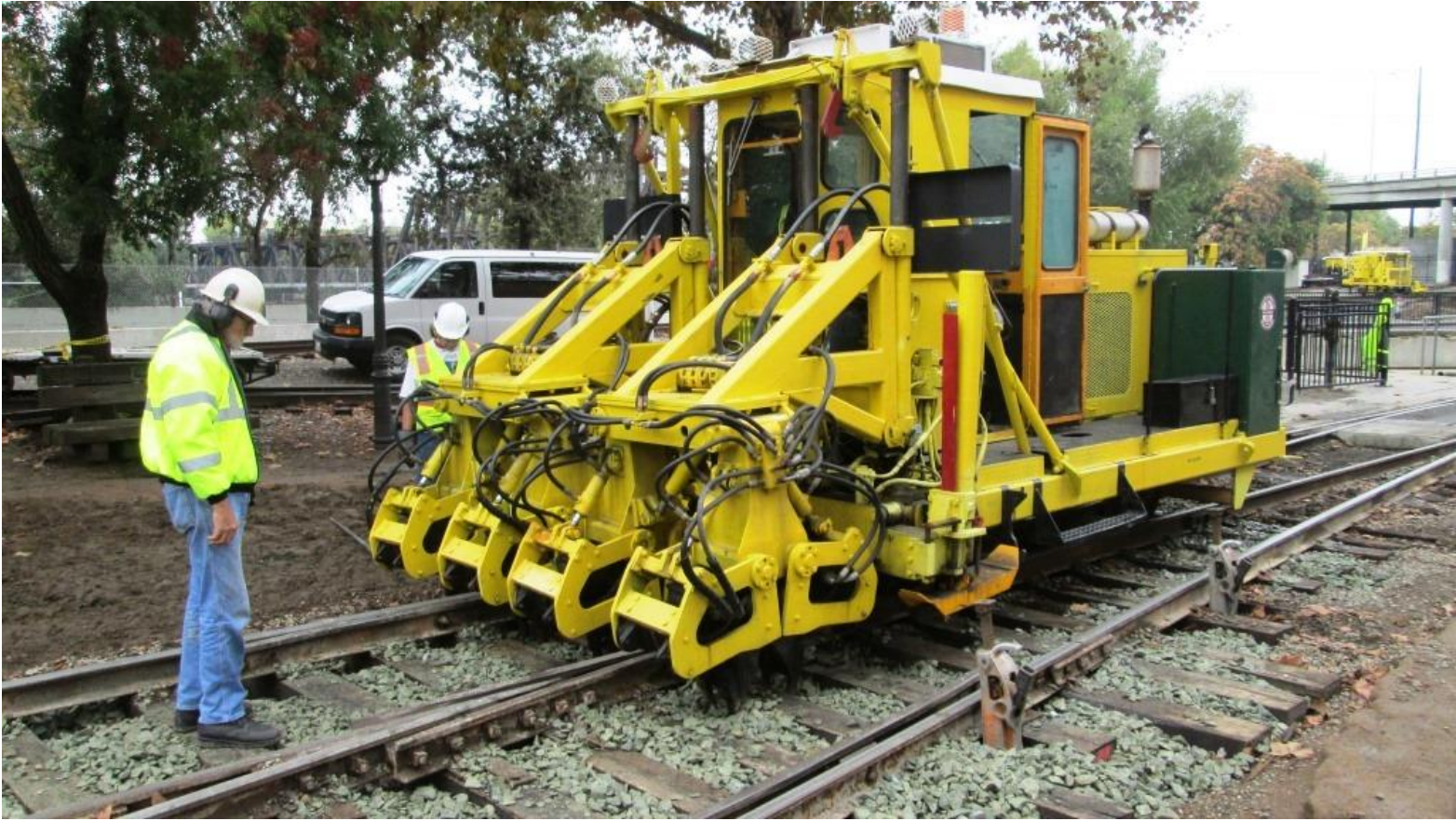
The tamper tamps rock under the ties
