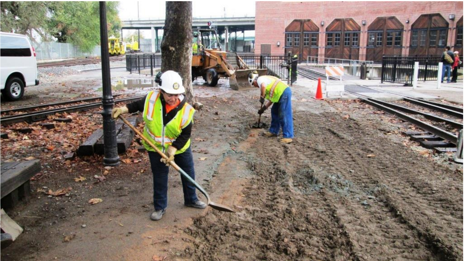
Pam and Clem do some clean-up work to the west of the Switch 1 Turnout
