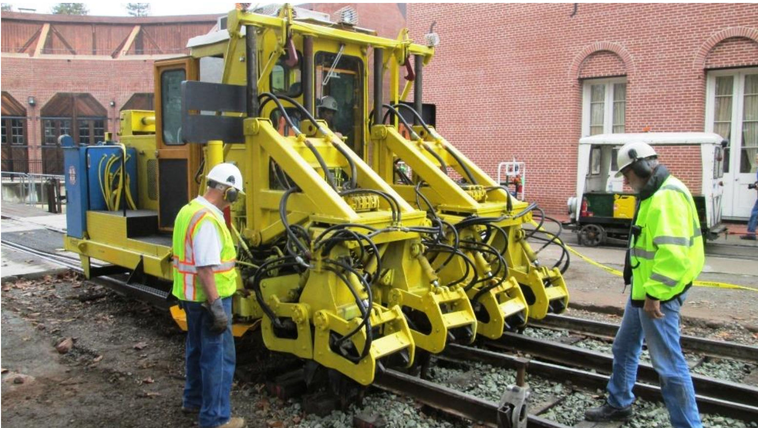
Clem and Alan work with Pam in the tamper to tamp around all the diverging rails
