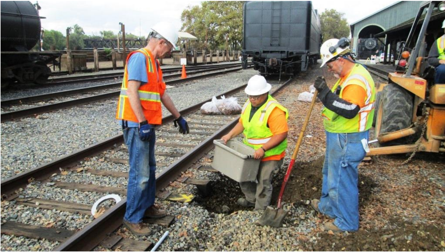
Dennis directs the placement of the electrical vault which Anthony sets in the ground
