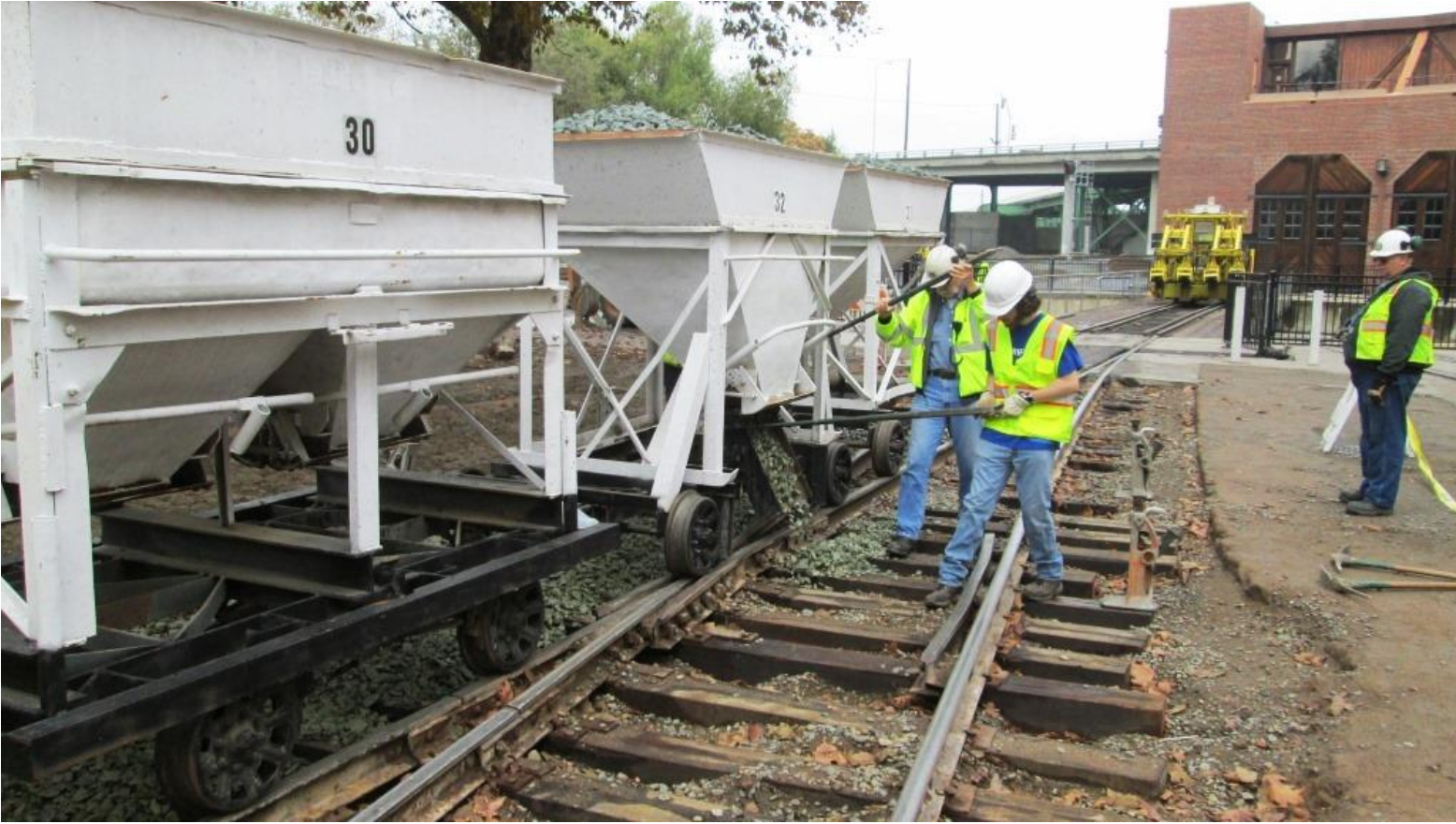
Alan and Matt continue the ballasting work
