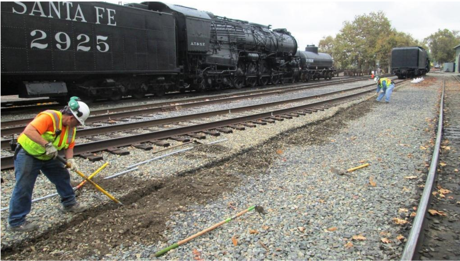
Joe and Heather continue digging the trench north along the Center Siding adjacent to the CPFD
