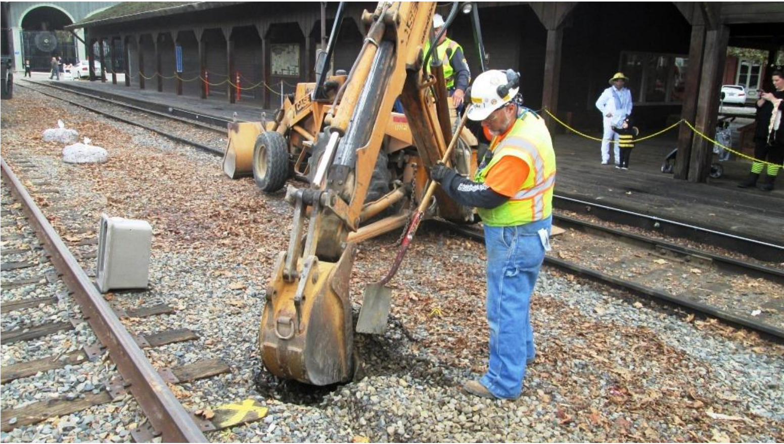
Mike F. breaks-up the clumps as Harry digs a hole for the electrical vault
