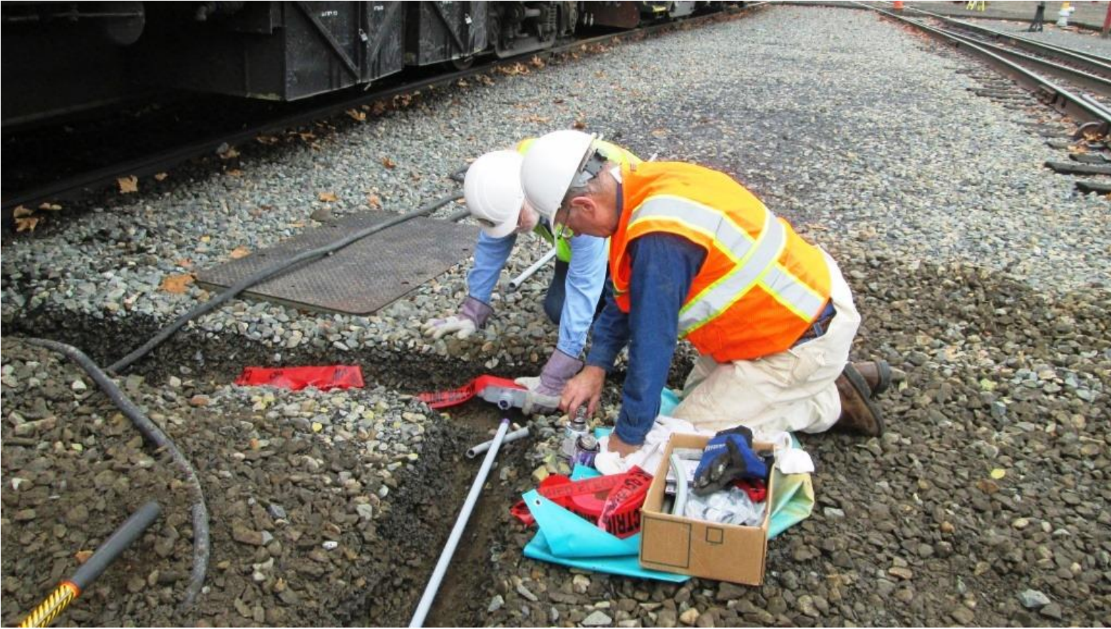
Carl and Dennis splice-in a junction-box
