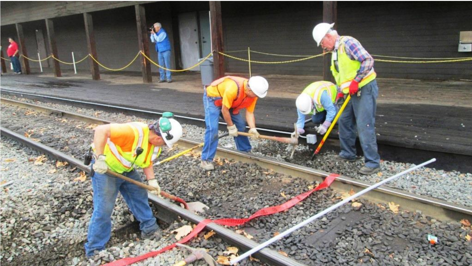
Joe, John, and Gary dig the trench from the junction-box under the Platform Track
