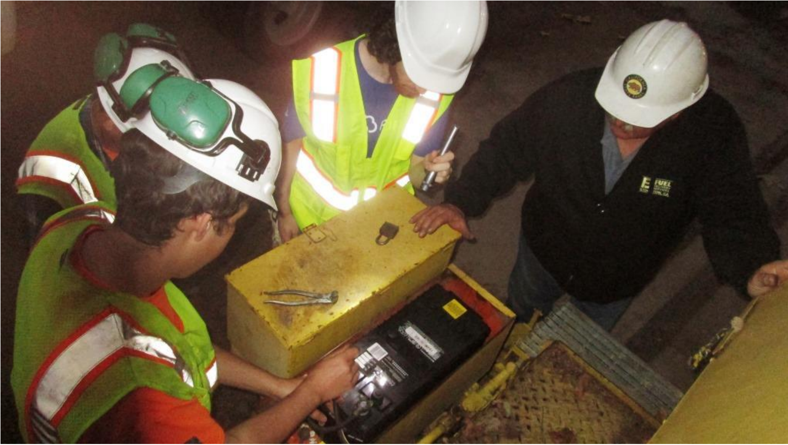
Weston, Joe, Matt, and Harry get man-lift's battery installed
