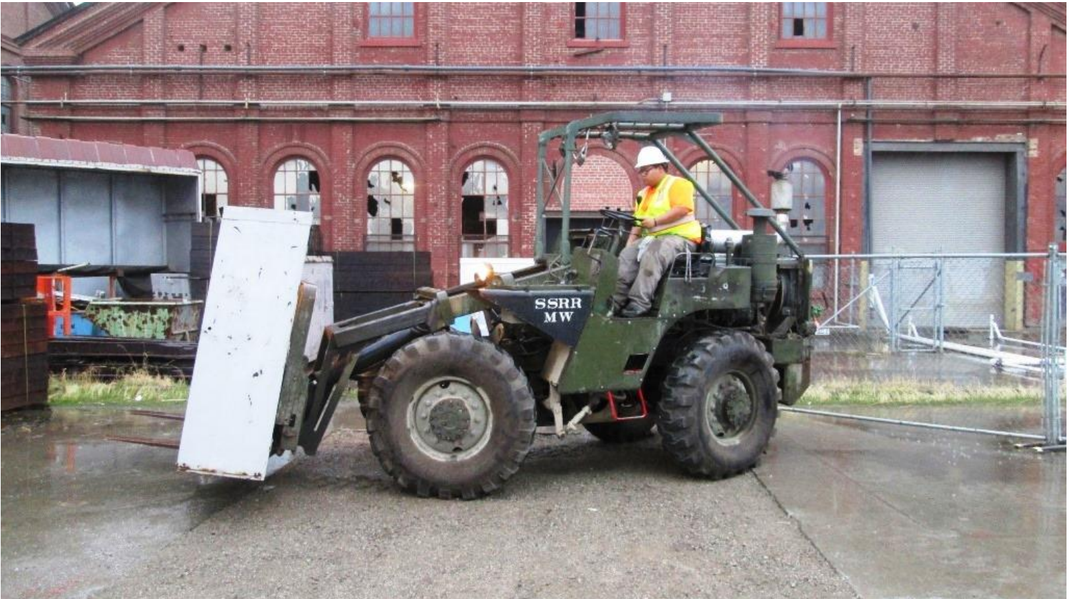
Anthony on Big Green takes a signal cabinet over to the Boiler Shop...
