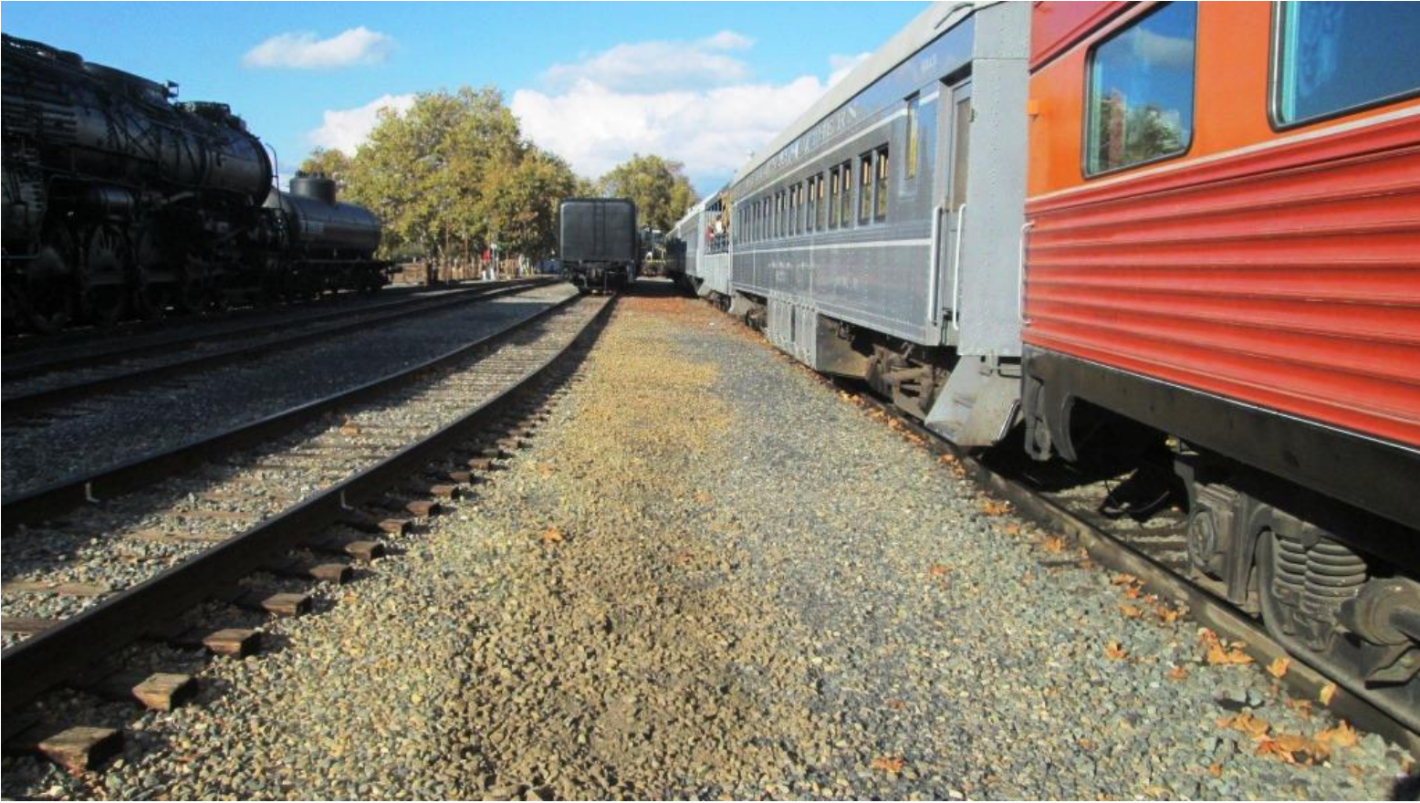
At day's end, one could hardly tell that any ground had been disturbed at all
