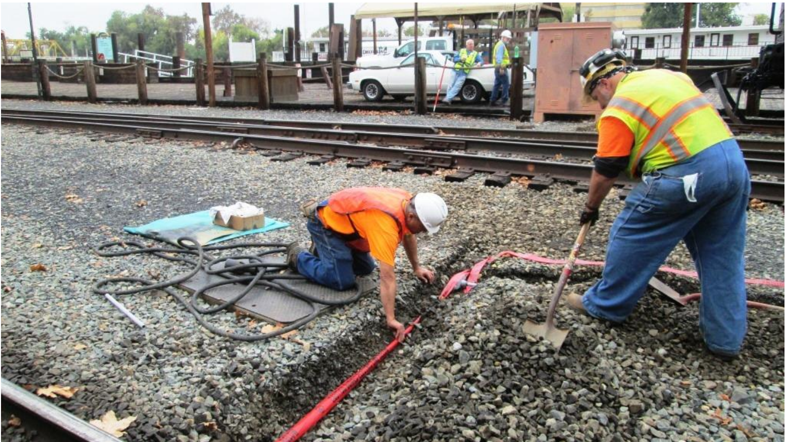
John covers the conduit with red warning tape as Mike F. begins filling in the trench
